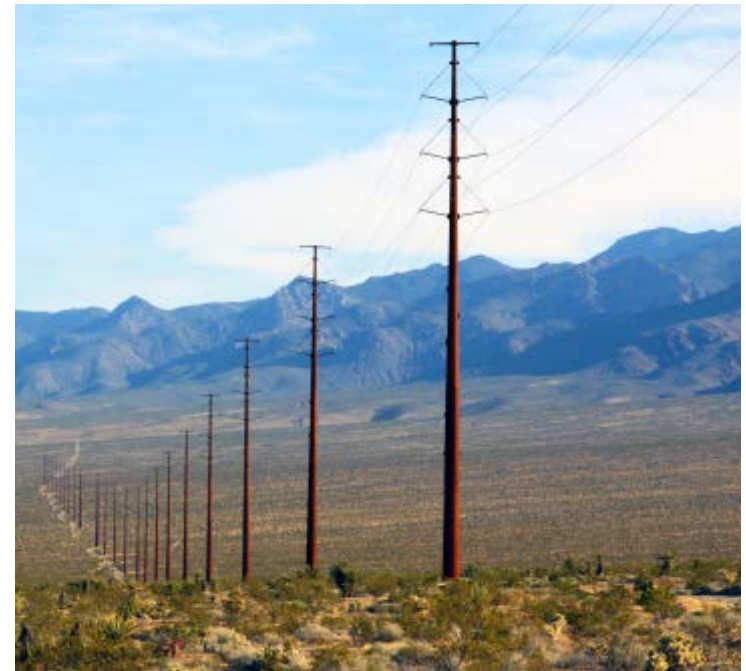
GridLiance West Transmission System
